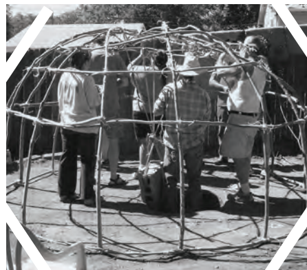
The traditional Native sweat lodge is made of willow branches tied together and covered with natural materials that "breathe."
